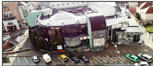
100m 2 of BIPVs (Glass) on the Glass Façade of Alba Iulia Municipality Building (Romania)
